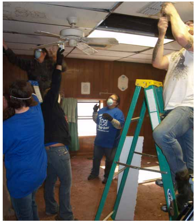
While some workers ripped up carpet and carried out insulation, left, others worked on ceiling tiles and wiring, above.
